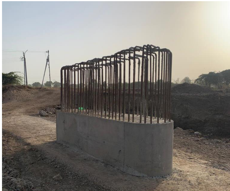
Figure 1.1: Partially completed column structure of NH-6
