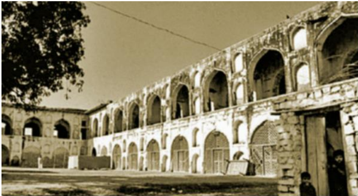
Dar-ul-Shifa (House of Cure), A building with arches and a courtyard
