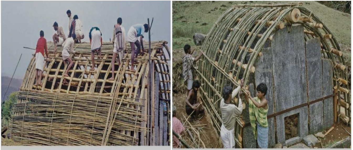
Construction of Arsh / Hut
