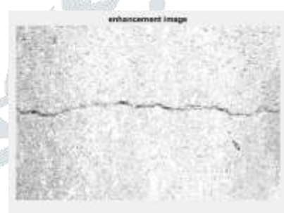
Fig20: Enhanced Crack Image
