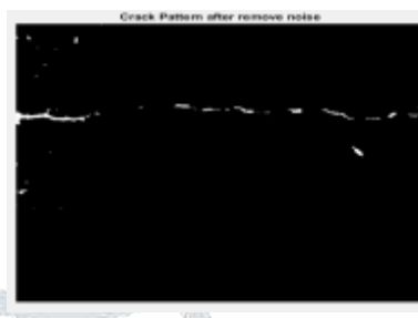
Fig24: Clear Crack Pattern After Removing the Noise.
