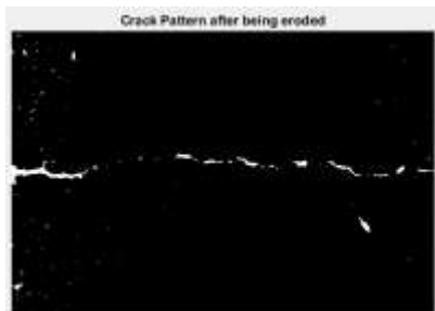
Fig23: Extracted Crack Pattern after being eroded.
